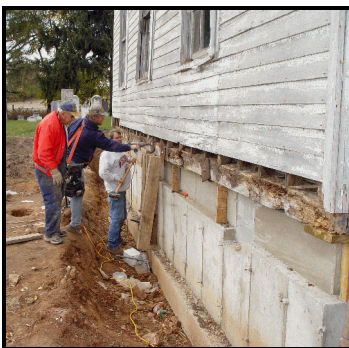
Myron Bacon, Tim Lipke and Mike Schmudlach aligned the building on the new foundation.
