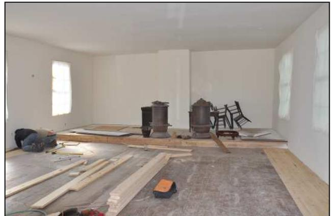
Workers finish restoring and strengthening the wood flooring on the 158-year-old structure.
